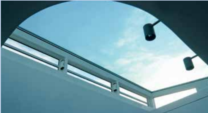
Horizontal installation of a large double glazed pane, e.g. for executive-standard private residential construction
